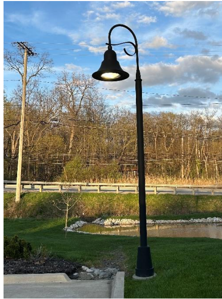
Figure 604-B – Cut-off light fixture example
